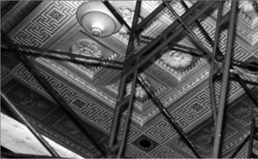
Image 4: A section of the light-blue color scheme on the Courtroom ceiling and one of the old pendant lights, seen through scaffolding during repainting, early 1970s. Collection of the Supreme Court of the United States.
